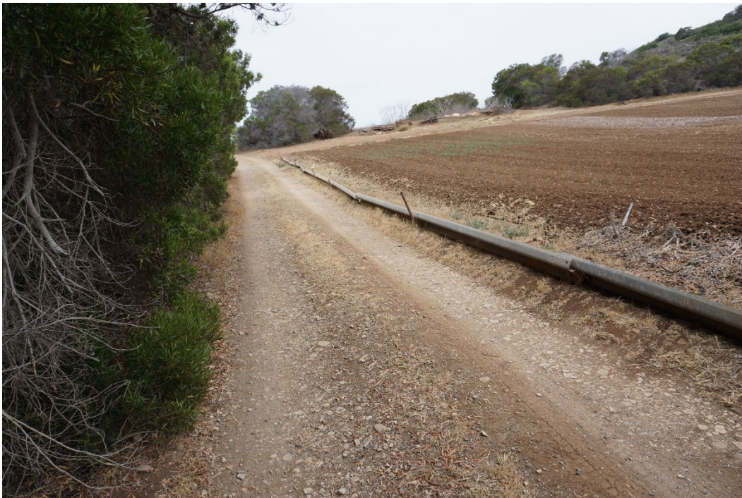
Photograph 10. Vehicular road. View facing southwest. July 26, 2022.
